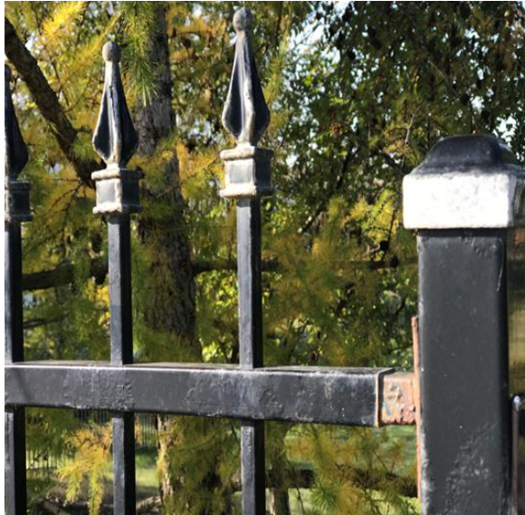
Repaired and prepared aluminum fences for painting
